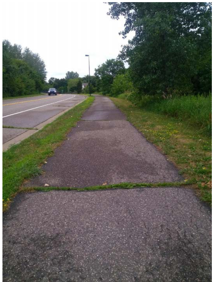
Figure 3.18: An example of an Oakdale shared use path along Helmo Avenue that would benefit from crack and surface treatments.
