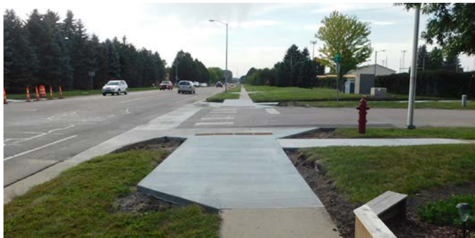
Figure 3.4: This image of an ADA ramp replacement project in Brookings, SD illustrates how an intersection project can be designed to prepare for a future shared use path project along the entire street.
