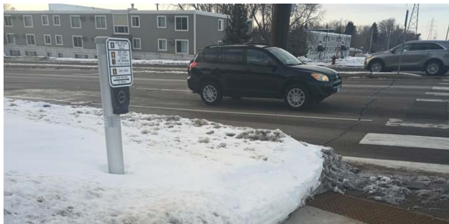
Figure 3.16: A wintertime access route to a pedestrian push button is needed at this intersection on Hadley Avenue at 10th Street (left), while a maintained sidewalk is needed at this transit stop also on Hadley Avenue just south of 10th Street (right).
